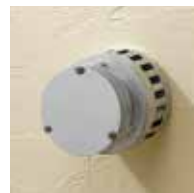
Balanced Flue (No chimney required)
