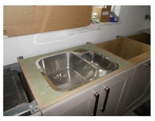
In an 800mm or wider unit, the sink to be set into a piece of MDF or similar, supported within the unit.
