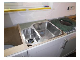
In a 600mm wide unit, the sides of the carcass to be routed out to let the flange of the sink in.
